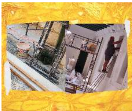
Maintenance being carried out at college
